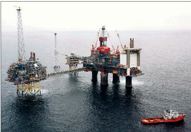
Burial at sea. A million tons a year of CO 2 from the Sleipner natural-gas field in the North Sea are reinjected underground.
